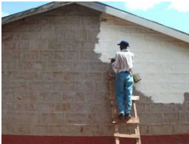
Artist Maina preparing the wall with undercoat paint
