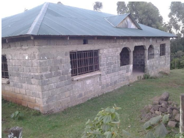
The resource centre under construction.
